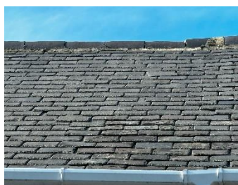
Pic 9 and 10 : slipped slates
