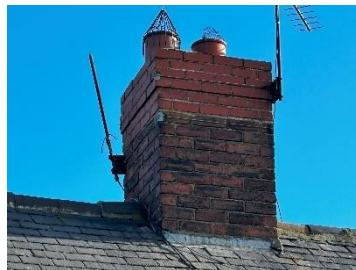
Pic 6: Chimney Rear elevation
